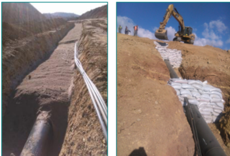
Figure 3-7: Procedure for backfilling the pipeline trench
