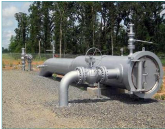
Figure 3-17: Pig Launcher surface facility
